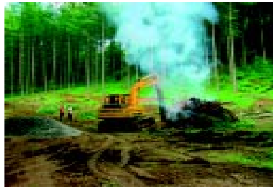
Great Wood Car Park work starts in 2001
